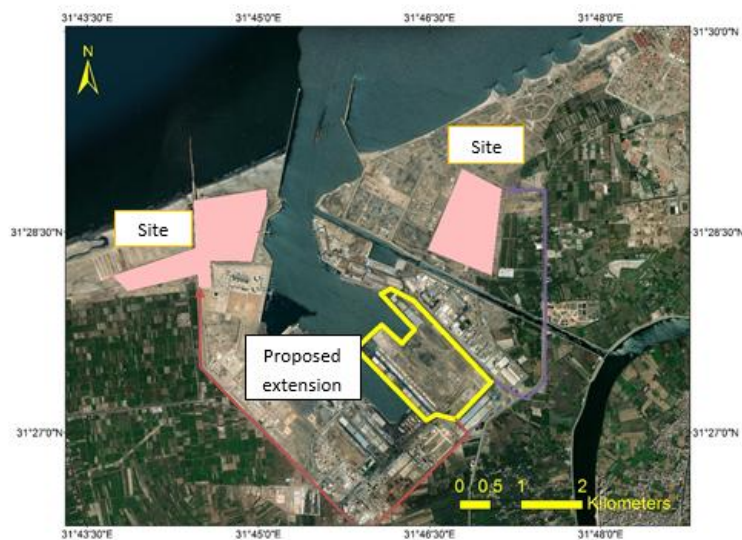
Fig. 21. Two sites proposed to dispose sediment dredged from the extension harbor basin (project area)
