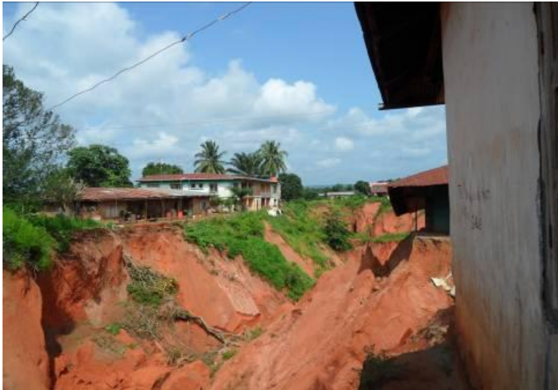
Fig. 7. Buildings about to be swallowed by gully erosion in Auchi
