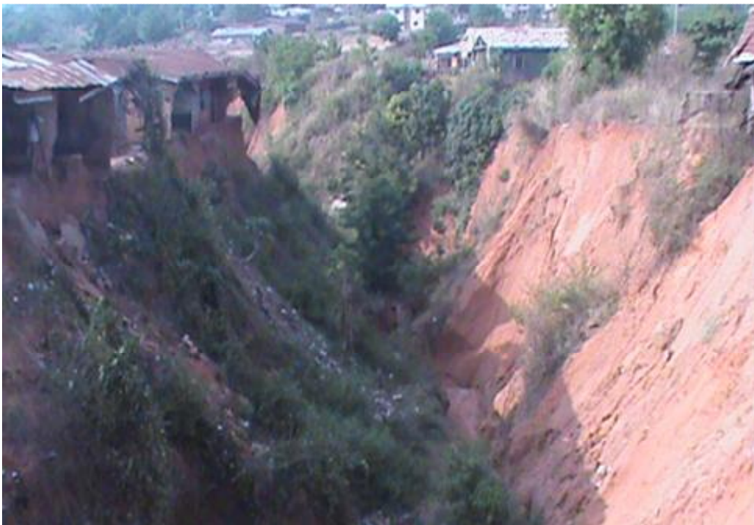
Fig. 9. Buildings under the threat of gully erosion in Auch
